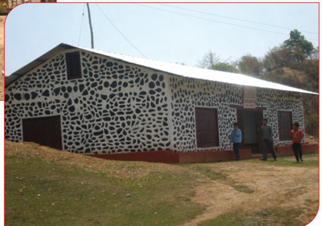
Chapakhori SHP Building: During & After Renovation, Kavre
